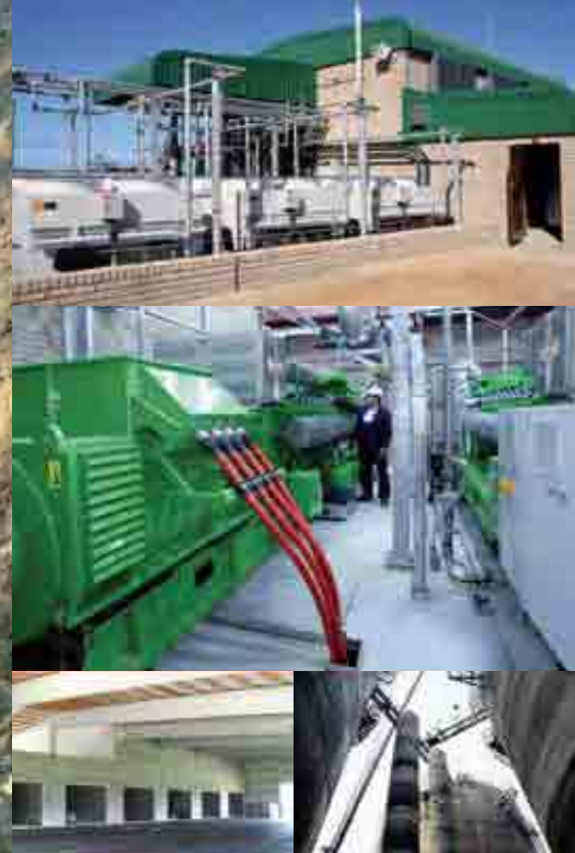
Clockwise from above left: Reinforcing of the Digester in progress at Cato Manor, South Africa; The biogas power building and 1.416 MW Jenbacher gas gensets at Petro SA; Dry fermentation energy recovery plant in Moosdorf, Germany; Bran Sands Waste Water Treatment, UK.
