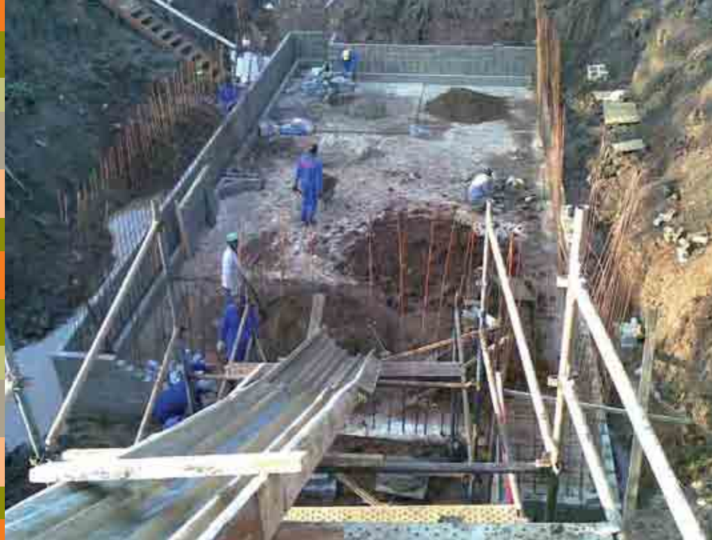
Clockwise from above left: Reinforcing of the Digester in progress at Cato Manor, South Africa; The biogas power building and 1.416 MW Jenbacher gas gensets at Petro SA; Dry fermentation energy recovery plant in Moosdorf, Germany; Bran Sands Waste Water Treatment, UK.
